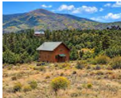
View of Cabin
